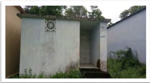
Common Toilet at Tangi Range of Chillika Wildlife Division (APO Year – 2012-13)
