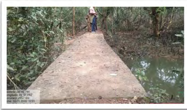
Culvert at Kanika Range of Rajnagar Wildlife Division (APO Year – 2011-12)
