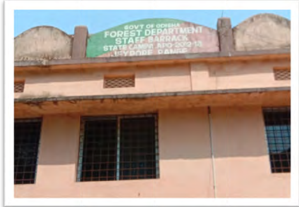
Staff Barrack at Jayapur Range of Jayapur Division (APO Year – 2012-13)
