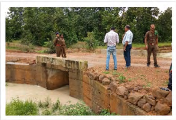
Culvert at Gopalpur Range of Sundargarh Division (APO Year – 2016-17)
