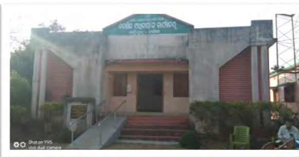
Range Office at Mahipur Range of Nayagarh Division (APO Year – 2012-13)
