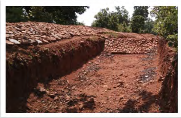
Graded Bund at Khalasuni Range of Bamra WL Division (APO Year – 2016-17)
