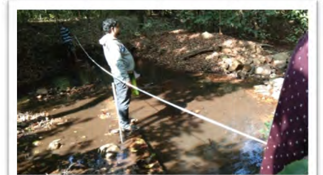
Surface Dyke at Kusanga Range of Mahanadi Wildlife Division (APO Year – 2016-17)
