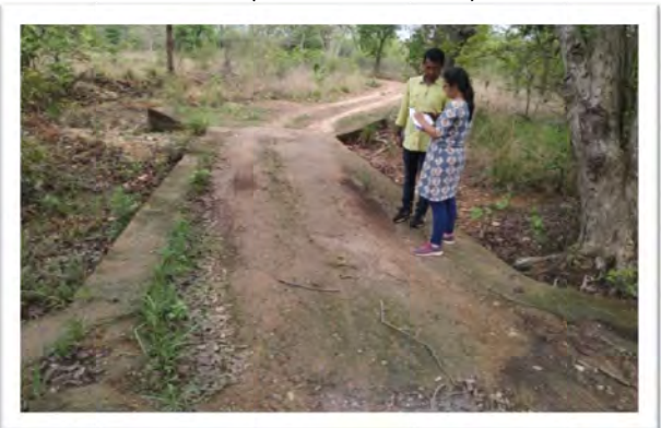
Causeway at Lakhanpur Range of Hirakud WL Division (APO Year – 2012-13)
