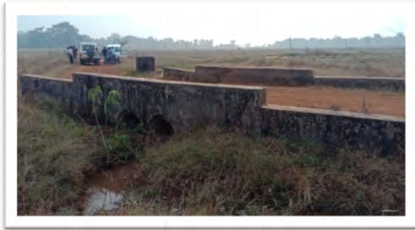
Culvert at Sukinda Range of Cuttack Division (APO Year – 2011-12)
