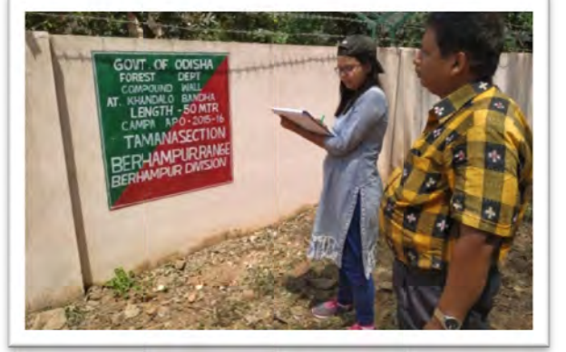
Compound Wall at Berhampur Range of Berhampur Division
