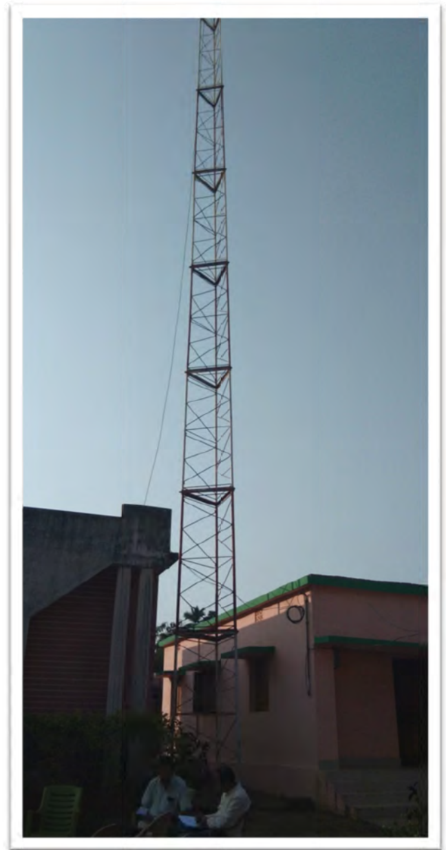
VHF Tower at Mahipur Range of Nayagarh Division (APO Year – 2016-17)
