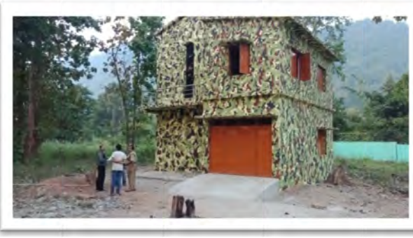
Staff Barrack at Purunakote Range of Satakosia STR (APO Year – 2016-17)
