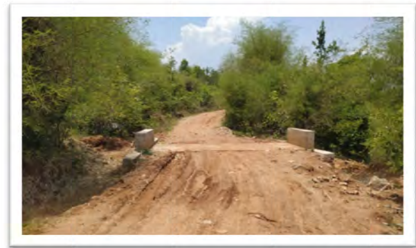
Culvert at Digapahandi Range of Berhampur Division
