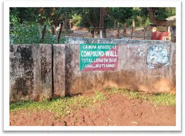
Compound wall at Khalikote Range of Berhampur Division (APO Year – 2012-13)
