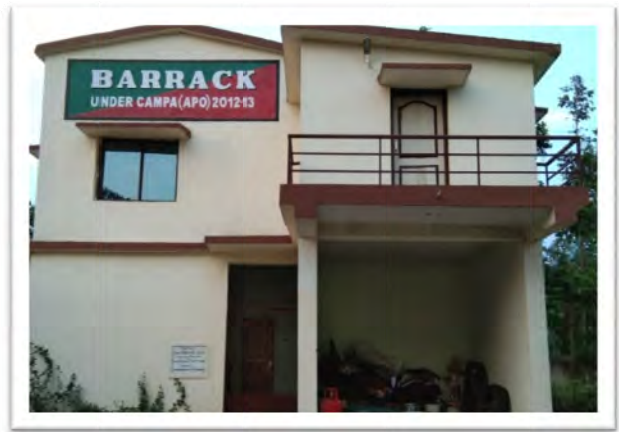
Staff Barrack at Rayagada Range of Rayagada Division (APO Year – 2012-13)
