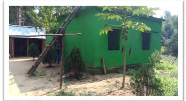
Antipoaching Shed at Pumpsara Range of Satakosia STR (APO Year – 2016-17)
