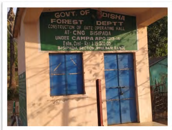
Gate Operating Hall at Phulbani Range of Phulbani Division
