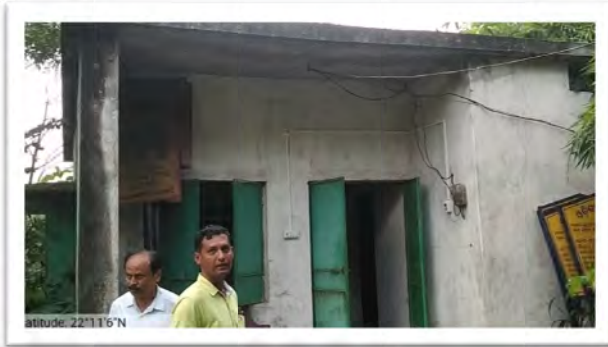
Labour shed at Kuanarmunda Range of Rourkela Division (APO Year – 2011-12)
