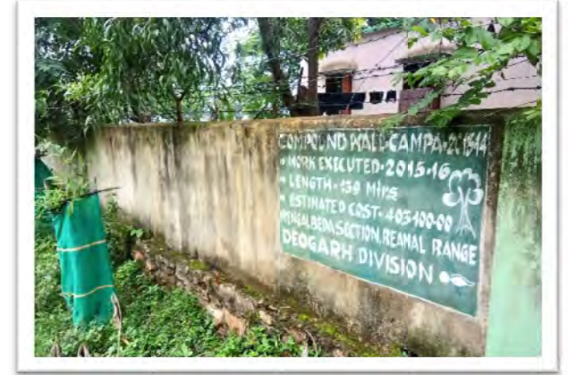
Compound Wall at Reamal Range of Deogarh Division (APO Year – 2015-16)
