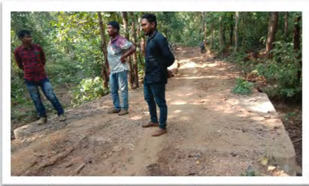
Culvert at Kesinga Range of Kalahandi North Division (APO Year – 2016-17)
